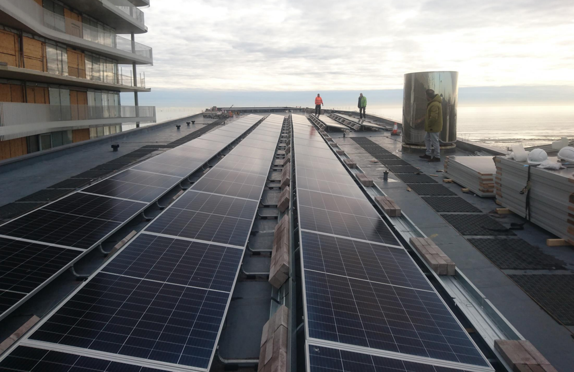
Brighton Energy Co Operative installing 100kW PV on Splashpoint, Jan 2020
