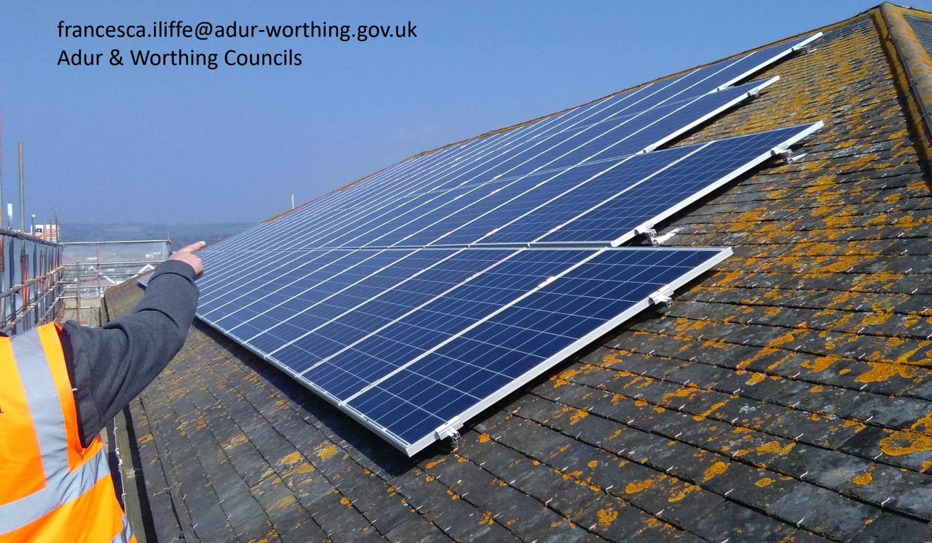
40kW PV array being installed on Portland House, 2017
