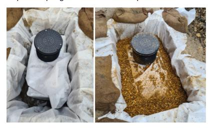
Step 3 – depending where you have installed refill hole and replace top surface. This is on a drive so was filled with hardcore and concreted. Now you can insert you sump pump and pump out whenever the need arises. The water can be recycled for watering lawns etc.
