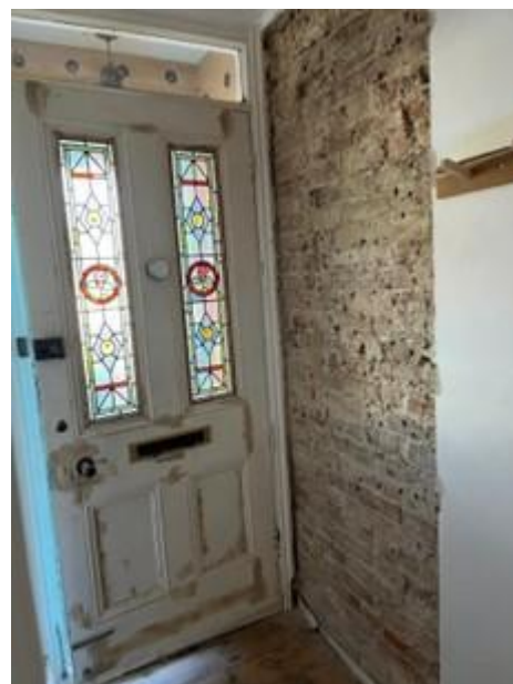
Plaster removed and Internal insulation added to prevent thermal bridging
