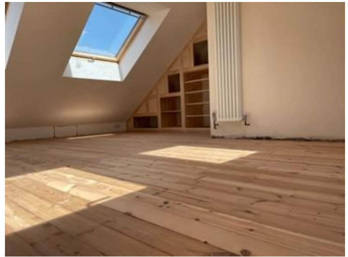
Woodfibre insulation, triple glazed Velux, floor made from rafters
